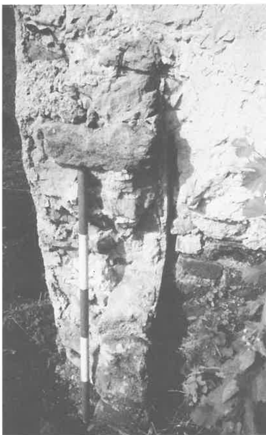
Abb. 11: Baufuge Pavillon–Nordmauer
